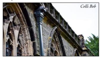
Finally some external works have been completed including lead roofing being sealed on the North aisle to prevent the current water ingress and the restoration of the hoppers and downpipes which are now looking fabulous, resplendent in their new grey paint.
