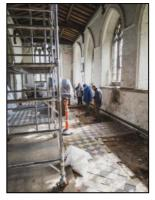
Scaffolding has been erected in the middle of the church - this has been put up in order to take down the early 20th century plumbing that runs hot water across the church ceiling. Indeed the removal of this pipe and all the old plumbing (except the large cast radiators) is the next significant piece of work to be undertaken. This will then allow the installation of the underfloor heating system.
