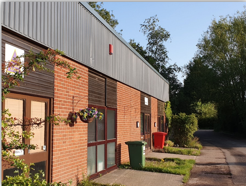
Figure 21: Willow Park Industrial Estate
